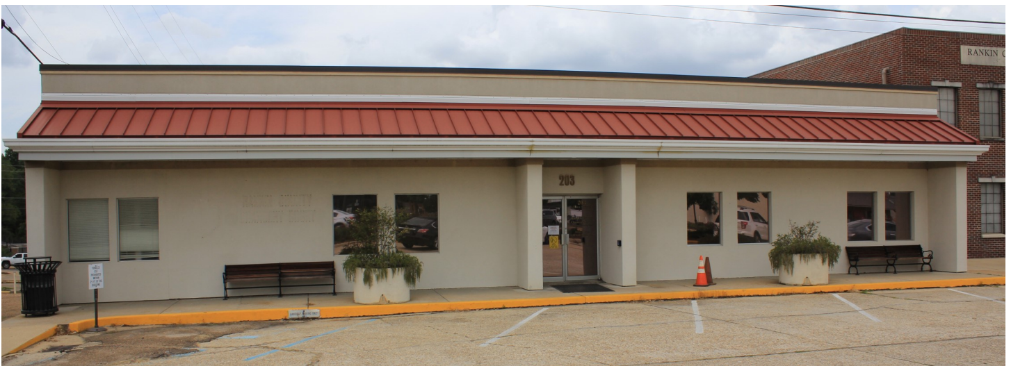
The old Rankin Chancery Building in Brandon was originally a grocery store. It will be renovated to house county offices.
